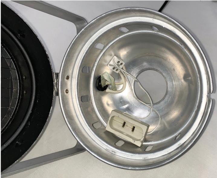
Front Screen in PAR Can to Secure Lotus LED Lamp in Place
